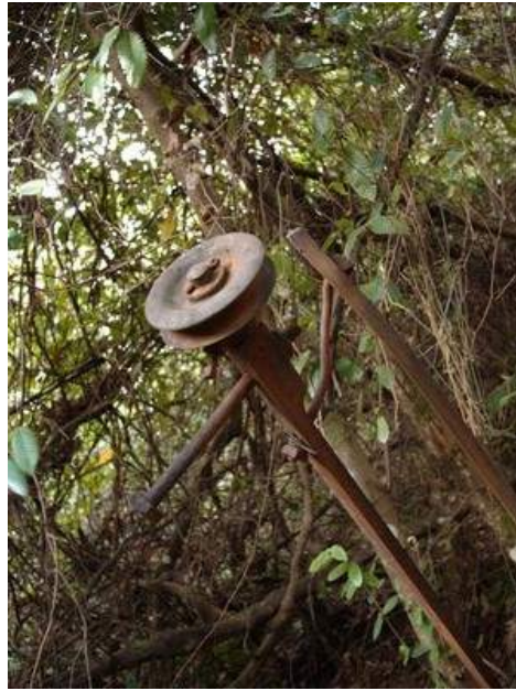
Figure 4.17 Wheel of track crossbar. (Photo: P1070508)
