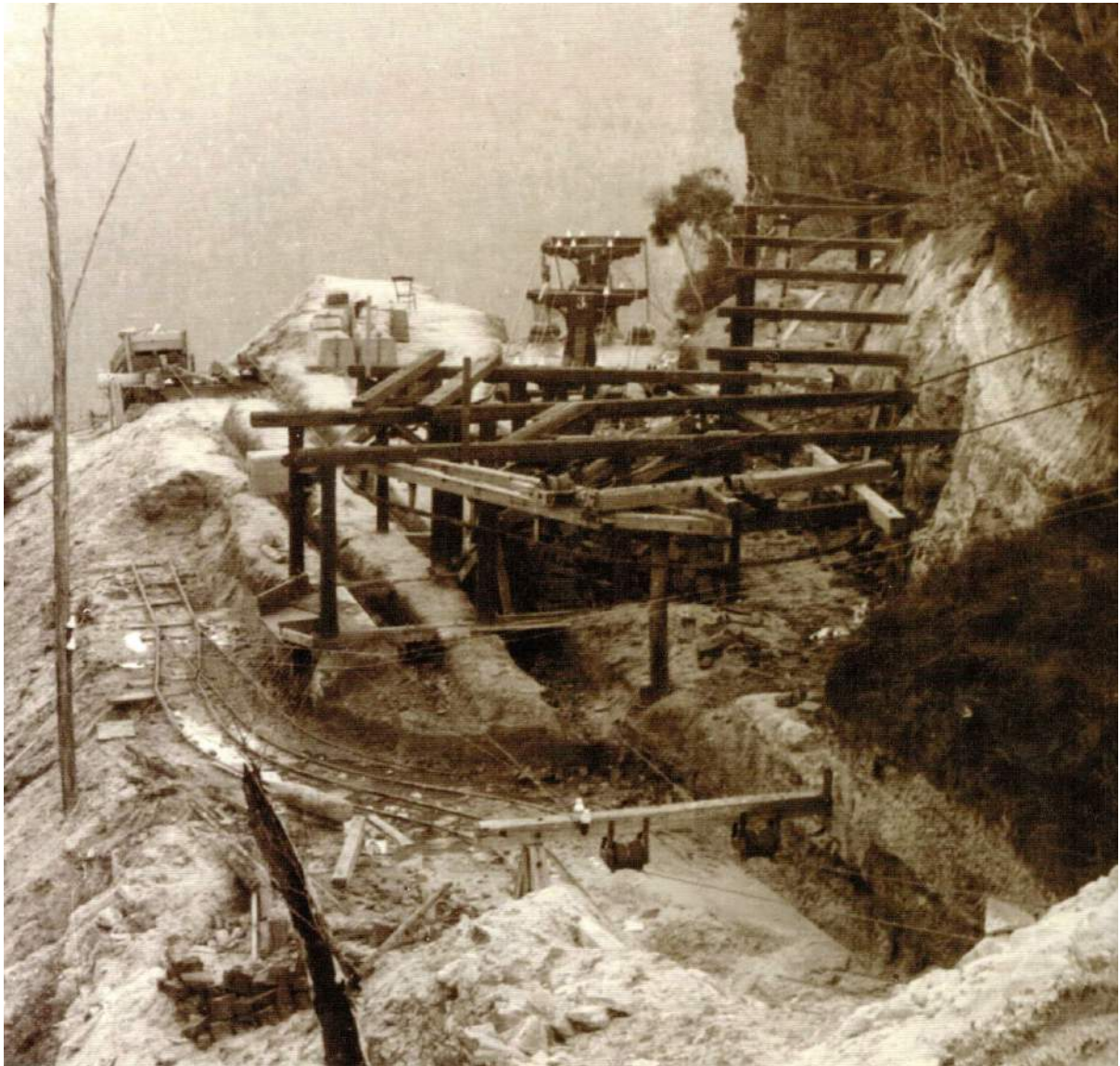
Figure 2.3 Northern unloading terminal of the ropeway. The number '3' can be clearly seen on the first tower. (Source: MacLeay Museum Sydney, original stereo photograph by Henry King, copy held by Blue Mountains Historical Society, reproduced in Pells & Hammon 2009: 86)
