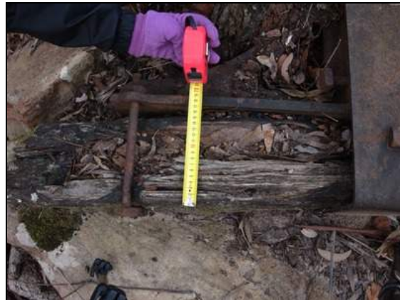
Figure 3.3 Measuring bolts in situ. (Photo: P1020051)
