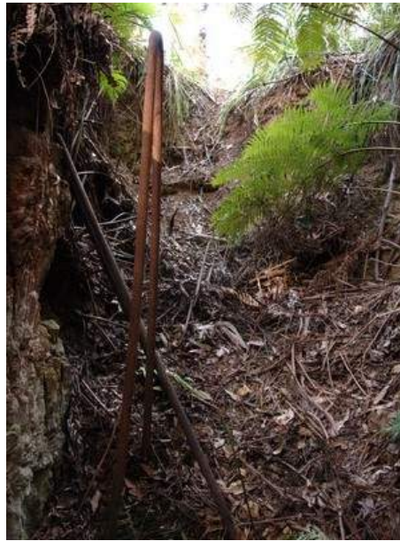
Figure 4.25 Detail of counterweight cradle in the base of the tension pit. (Photo: P1070471)
